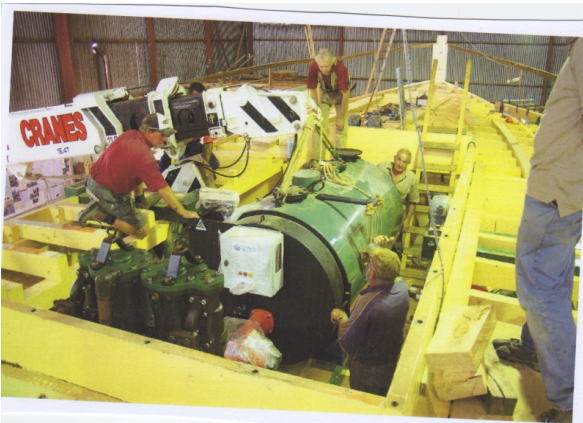
The engine being lowered into position
