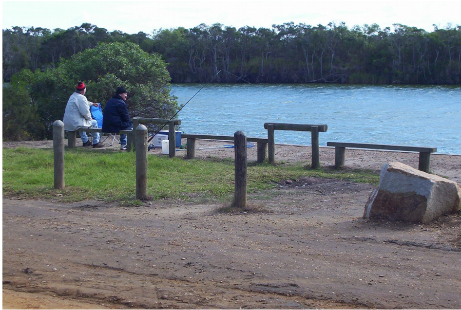
An example of a good Fishing Jetty on the Mitchell River but who constructed it and who financed it?
