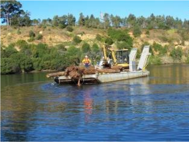
Photos show moving logs into position on the Nicholson River and Logs submerged
