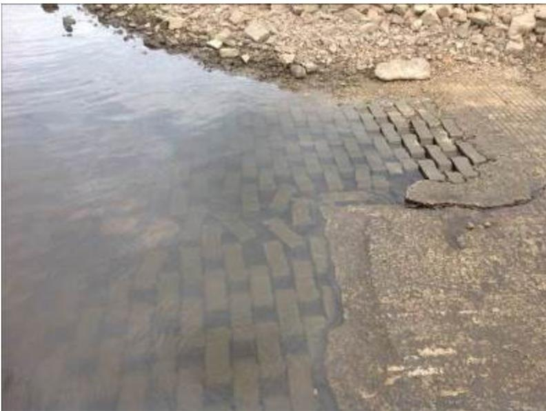
Sydenham Inlet opened just before Easter, and as expected the condition of the boat ramp has deteriorated. Large gaps between the concrete blocks are showing, (see attached photo) and care needs to be taken when unloading and loading of boats. A recent meeting with East Gippsland Shire indicated that repairs would be carried out soon.
